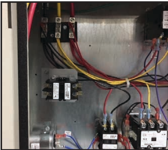
Figure 1. Contactor Location
