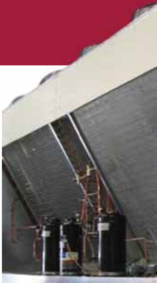
Dehumidification Circuit - Meets Standard 62.1 & 90.1
