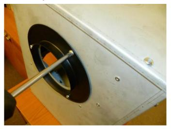
Step 2: Apply waterproof sealant apply to the inner face of the spigot along the line of the circle indicated.
