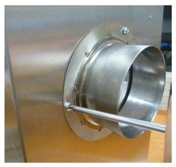
Step 4: Apply waterproof sealant to the mating surface along the line as shown in the picture below. Insert the wind and rain hood cover into the spigot.
