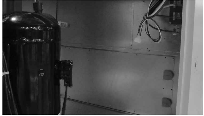
Figure 4. Electric Heat Access Plate
