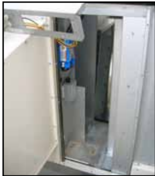
FIGURE 7 - Attach New Bracket to Re-locate the Display Module
