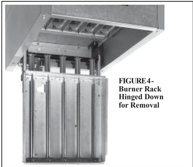
d) Allow the front of the burner rack assembly to drop down lifting up on the rear and sliding the complete burner rack assembly up and out of the manifold support brackets. The burner rack assembly should now be completely removed from the heater.
