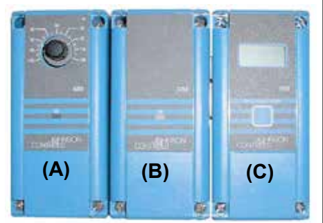
FIGURE 45 - Venter Speed Control Board in Control Options AG8, AG9, AG9H, AG40, AG58, AG60, AG61, AG62, DG1, DG5, D12B or D12C
