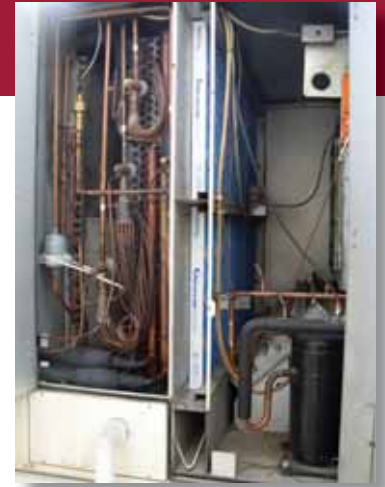
Dehumidification Circuit - Meets Std 62.1 & 90.1
