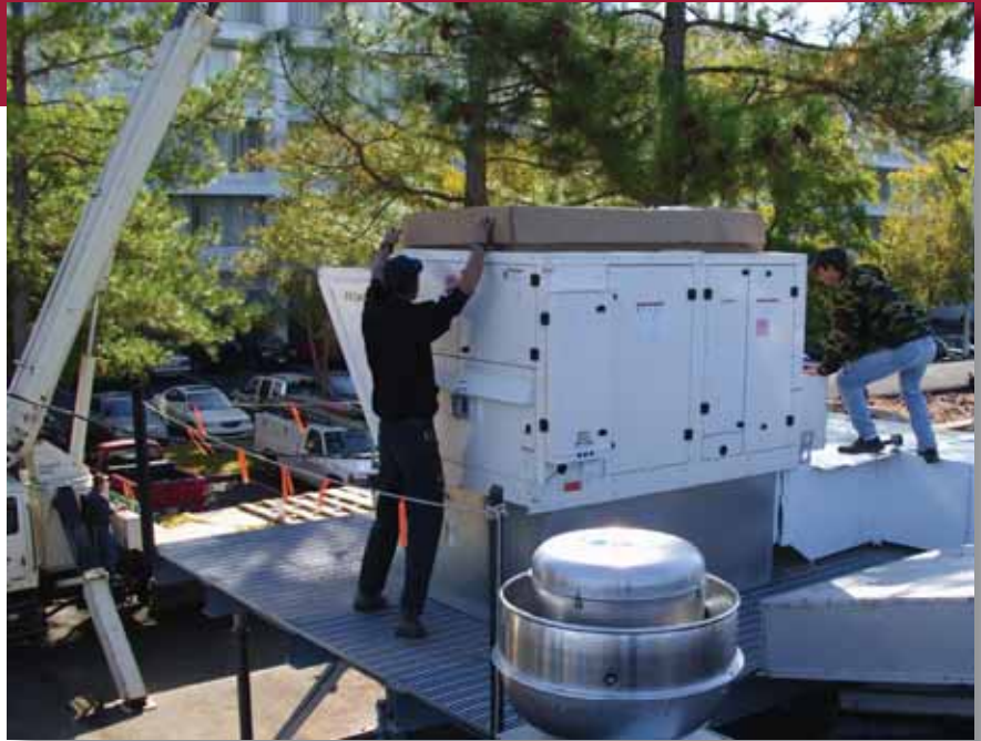
Kitchen Makeup Air and Space Temperature Control
