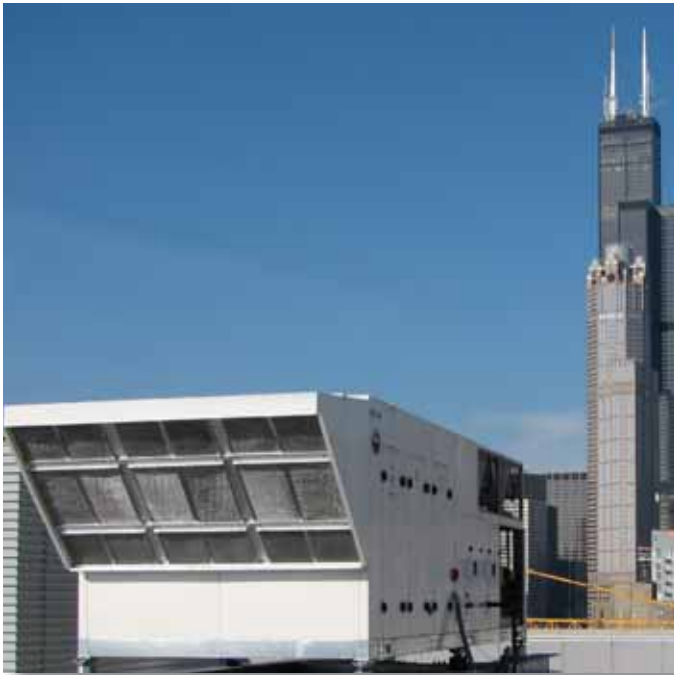
Condominium Corridor Makeup Air
