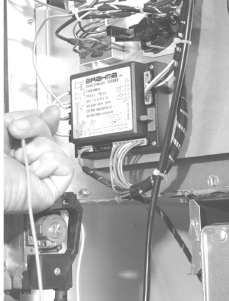
Figure 21 Disconnect wire of the ignition electrode at the burner controller
