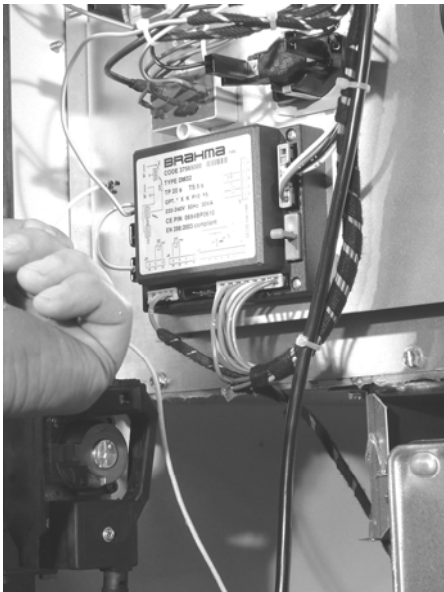
Figure 23 Disconnect flame sensor wire at the burner controller
