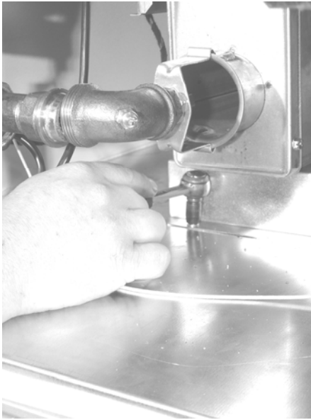
Figure 21 Remove 2 screws of the burner slider
