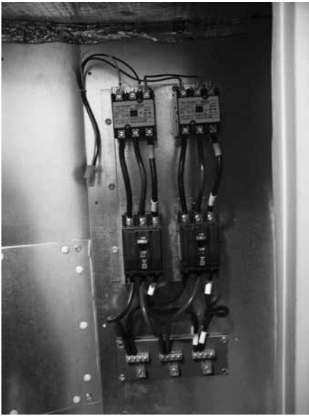
Figure 9. Circuit Breaker Mounting Plate Location
