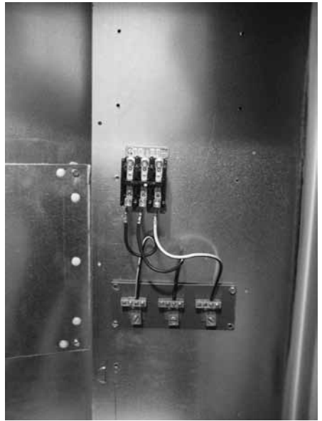
Figure 10. Single Contactor Mounting
