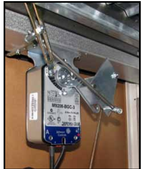
FIGURE 3C - View of Replacement Actuator and Linkage in a CAUA Mixing Box
