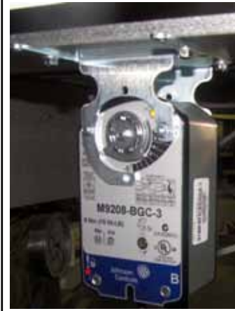
FIGURE 3B - Attach Replacement Motor and Crankarm
