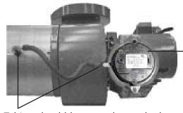
Pressure switch installed. Attach the black wire to the single prong and the orange wires to the 2-in-1 connection.
