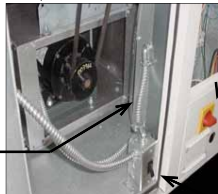
Factory-installed blower door safety interlock switch
