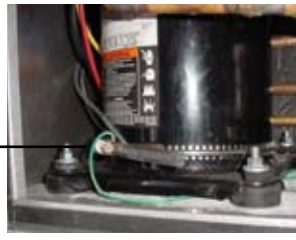
"Bellyband" Crankcase Heater
