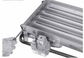
6. Install the drip shield screws to secure the drip shield. Reverse Step No. 2 on page 1.
