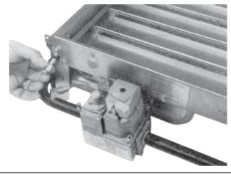
11. Install tubing and tighten. Leak test prior to placing unit into operation.
