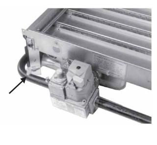
9. Install correct carryover orifice and brass compression fitting. See Step 10.
