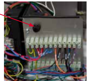
LC3 resetschakelaar Photon 25-100
